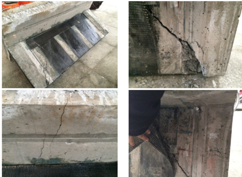
Fig. (8). The failure mode of Team DB-2.
