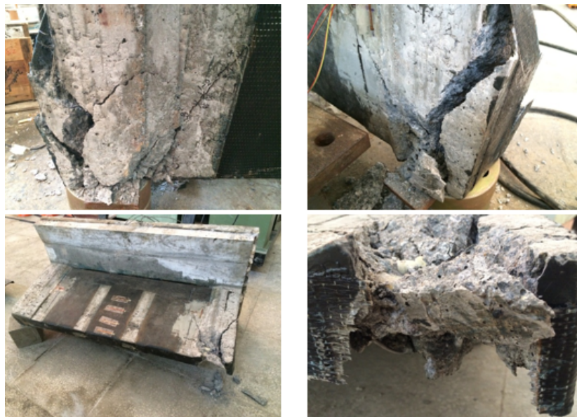
Fig. (7). The failure mode of Team DB-1.
