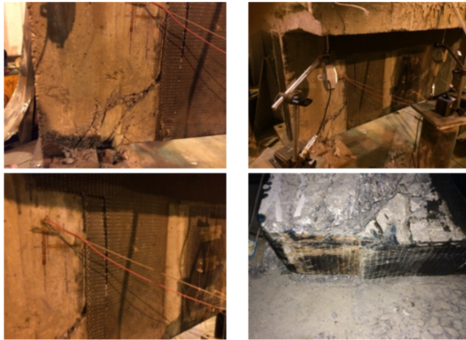
Fig. (10). The failure mode of Team YJG-2.
